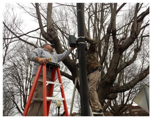
Each system will include a single 'Master transmitter" into which the music or audio will be fed. The Master transmitter needs to be within radio range of at least one of the pole-mounted units. It can even be located in an office somewhere on Main Street. Since the pole mounted units are "repeaters" the signal is propagated from one pole to the next and can even go around corners and down side streets, so the Master transmitter does not have to cover all units directly.
